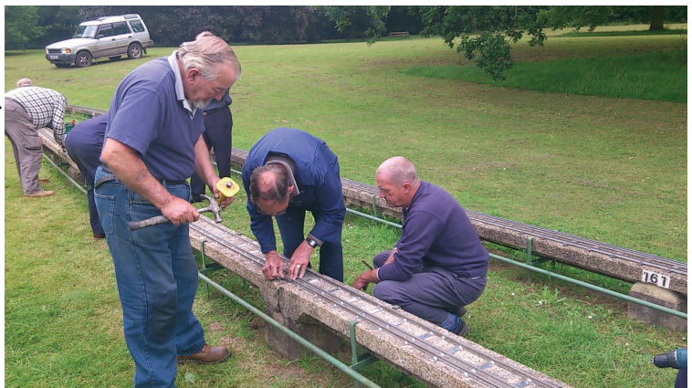
Almost there, the replaced track being readied for the first trains
