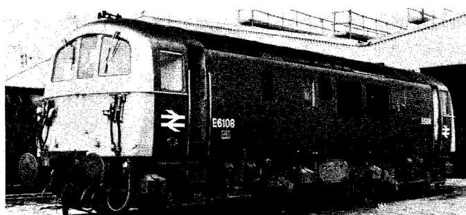
British Railways Class 74 750V d.c. electro-diesel Bo-Bo No. E6108
